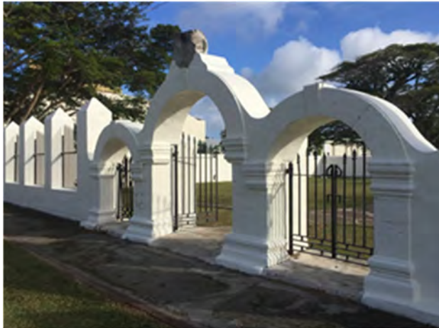
Iconic landmarks, like the arches of the Almacén, should be well-maintained and protected from alteration and deterioration.
