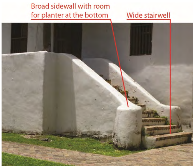
Example of wide stairwells.
