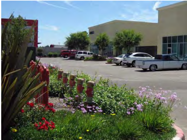
Landscaping screens these utilities and enhances the aesthetics of both these utilities and the overall site.
