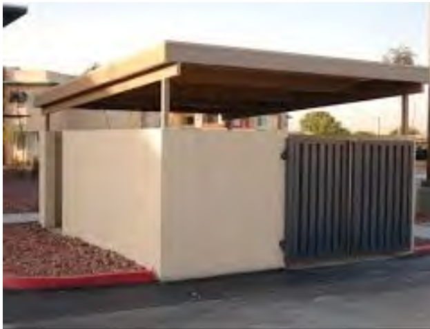
An example of an enclosed trash receptacle location that is compatible with the main building it is associated with. A roof
