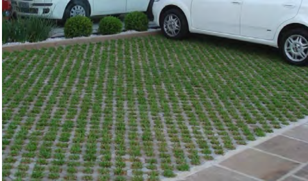
Example of a surface parking lot using grass pavers to help mitigate stormwater.
