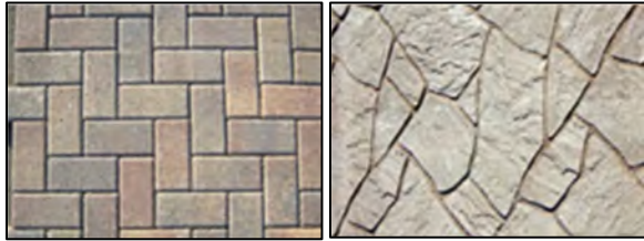
Examples of pavement textures, pavers (L) and flagstone (R).
